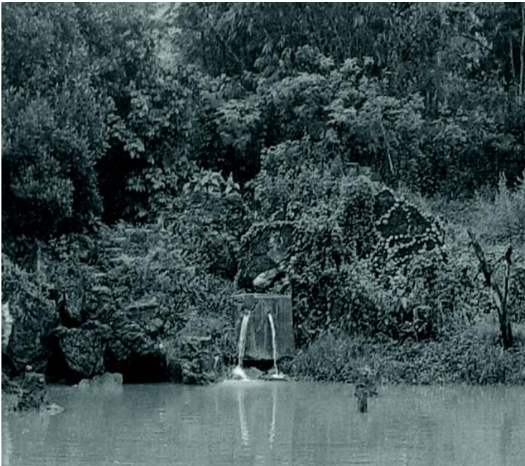
Cek dam Darunnajah 2, Cipining
